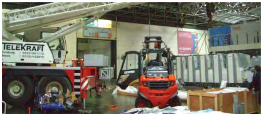
Heavy equipment makes installation a major task.
